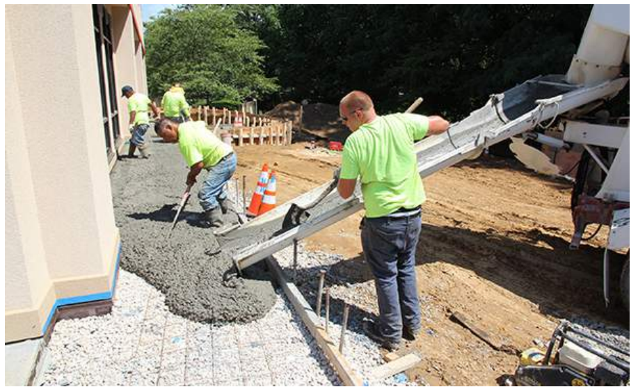
Workers pour and smooth out concrete along the southern side of the building.
