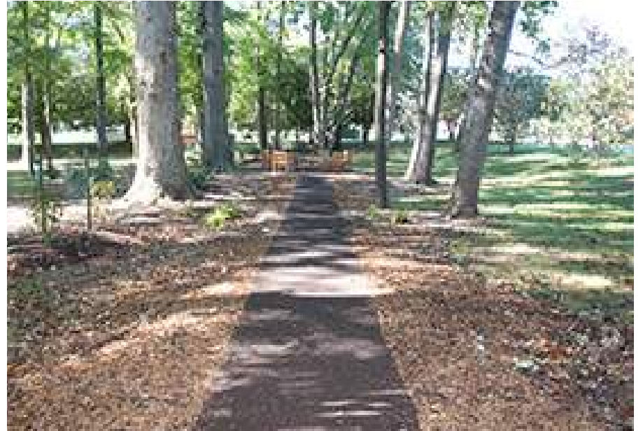
Above left, a rain garden in Mutual 7 helps manage stormwater runoff. Above right, porous pavement in Daffodil Park reduces stormwater runoff. Photos by Stacy Smith, Leisure World News
