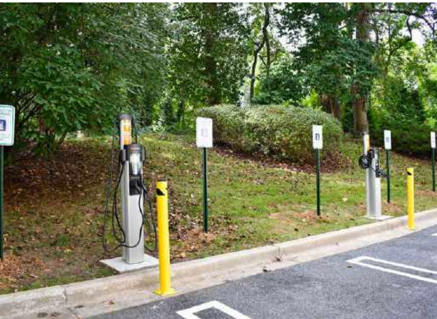
New electric vehicles charging stations at Villa Cortese, photo by Tim Carrico
